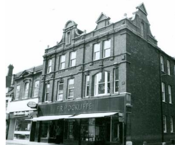
86 & 88 High Street, Bedford © Historic Environment Record, Bedford Borough Council
